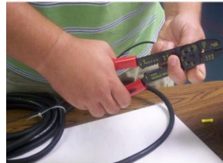
Figure 4.13 Strip 1/4" insulation
